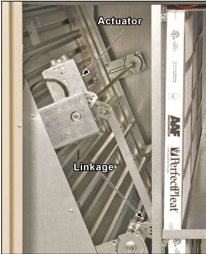
Figure 27: Damper Assembly
